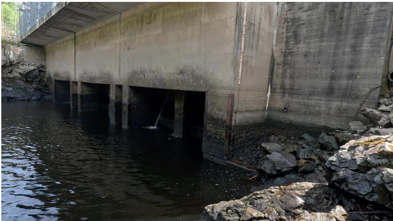
Figure 2, photo by Greg Sarnacki
