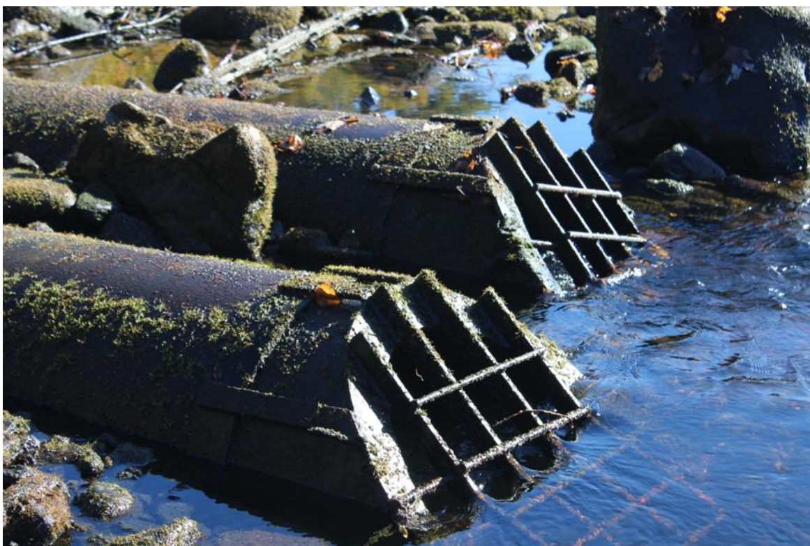
400 cfs provided adequate water to the intake pipes
